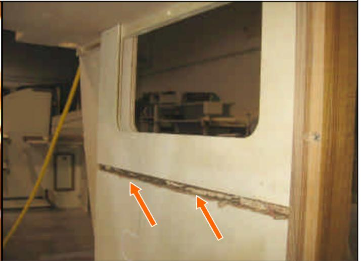
Fig.2 grind down screws that come out of receiver
