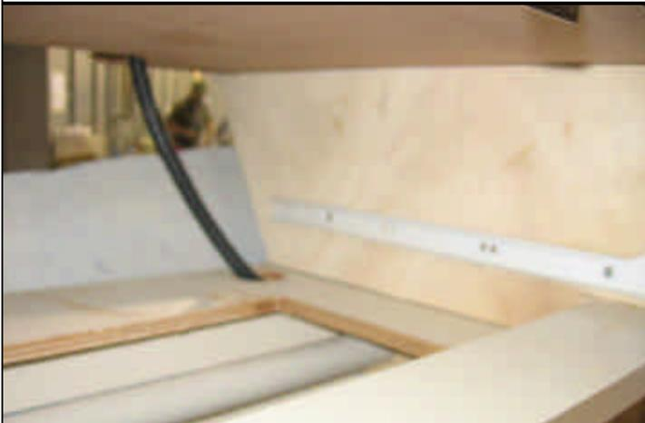
Fig.4 Pull the freezer wires from sub floor cutout, run the wires upward.
